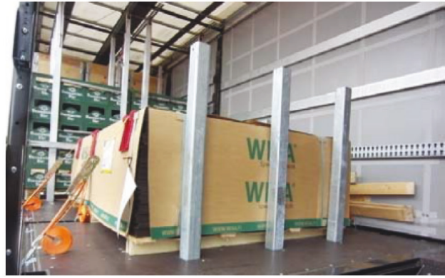
Figure 7: Stanchions used for blocking in forward direction
