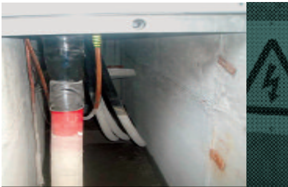
Fig 8.1 Termination of cables including high voltage cable
