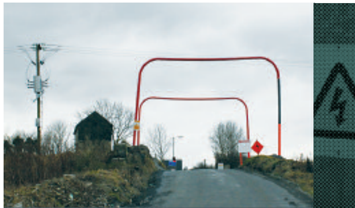
Fig 18.2 "Goal Posts" on traffic route to protect against contact with overhead line
