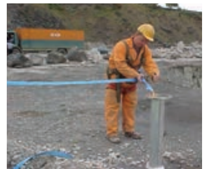
Figure 30: Installing quarry face edge protection
