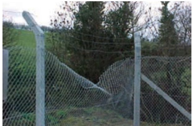
Figure 34: Protecting the boundary of a quarry from inadvertent access
