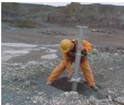
Figure 29: Installing quarry face edge protection
