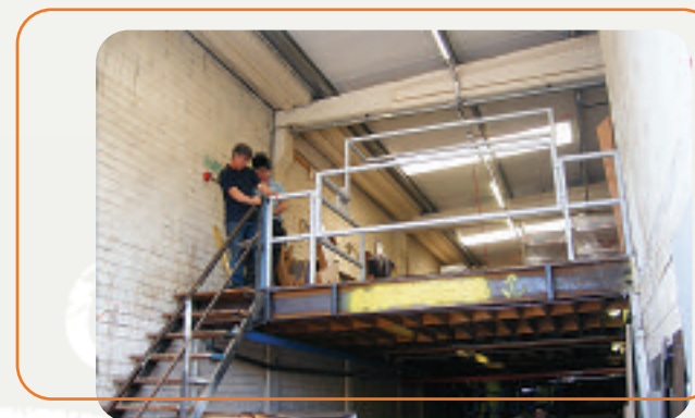
Figure 4 Fabrication of an up and over handrail
