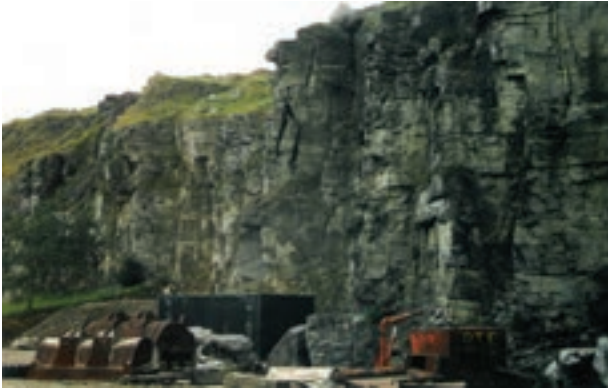
Figure 41: Significant Hazard – loose blocks above working area
