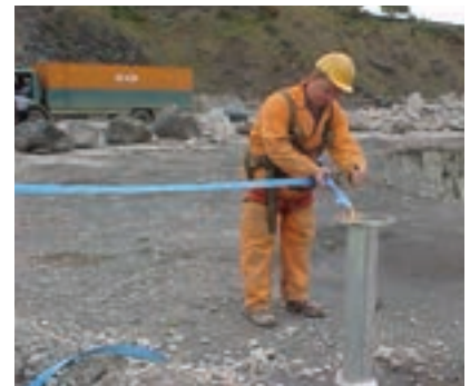
Figure 30: Installing quarry face edge protection
