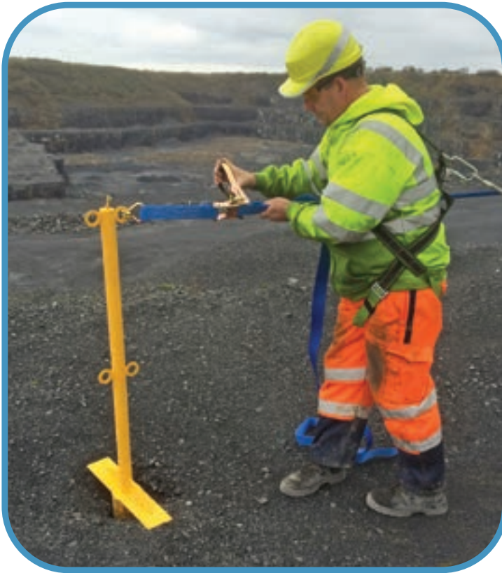
Strap and Pole system being erected and tensioned by a person using a harness with inertia reel lanyard
