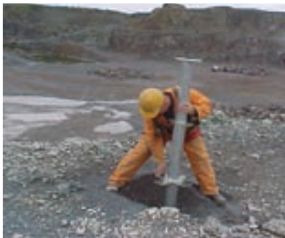
Figure 29: Installing quarry face edge protection
