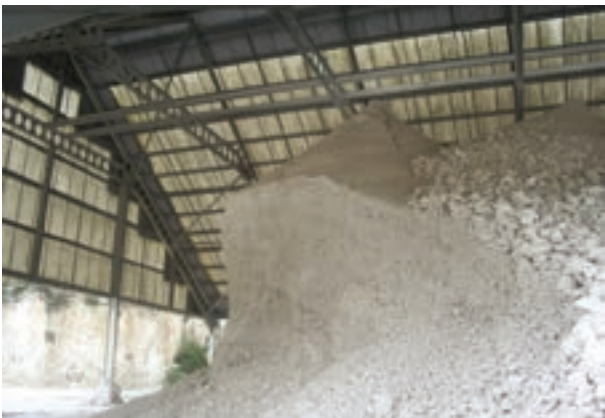
Figure 42: Significant Hazard – unstable stockpile recovery face
