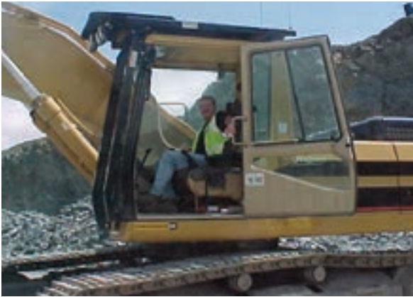
Figure 20: Excavator with falling object protection provided
