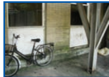
Asbestos cement wall panels
