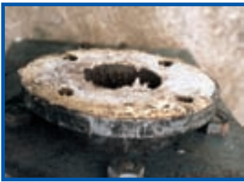
Exposed chrysotile-based compressed asbestos gasket to flange
