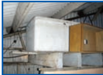
Asbestos cement water tank in attic
