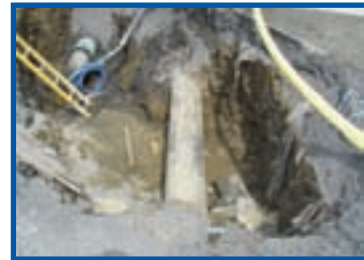
Asbestos cement water main
