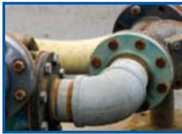
Compressed asbestos gaskets to pipework flanges
