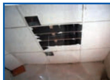
Damaged AIB ceiling panels
