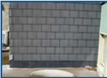
Asbestos cement flat profile roof tiles
