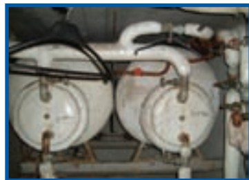
Thermal insulation to calorifier
