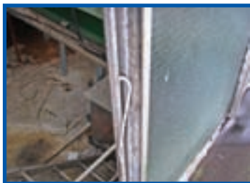
Chrysotile rope seals in glazing units
