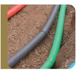
Telecommunications cables may be installed in concrete pipes, smooth black ducting or grey corrugated ducting. All cables should be assumed to be live until disconnected and proved to be safe. Contractors should obtain written confirmation of disconnection from the utility/service provider before removing a redundant service or arrange for the utility/service provider to remove the service.
