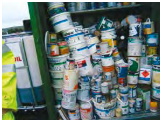
Figure 18. Inadequate storage of materials can lead to accidental spills.
