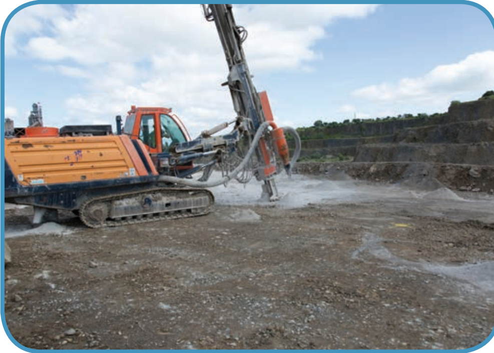
Drill Rig Operator working at a Quarry Face with fall protection provided by bunded edge protection made from quarried material
