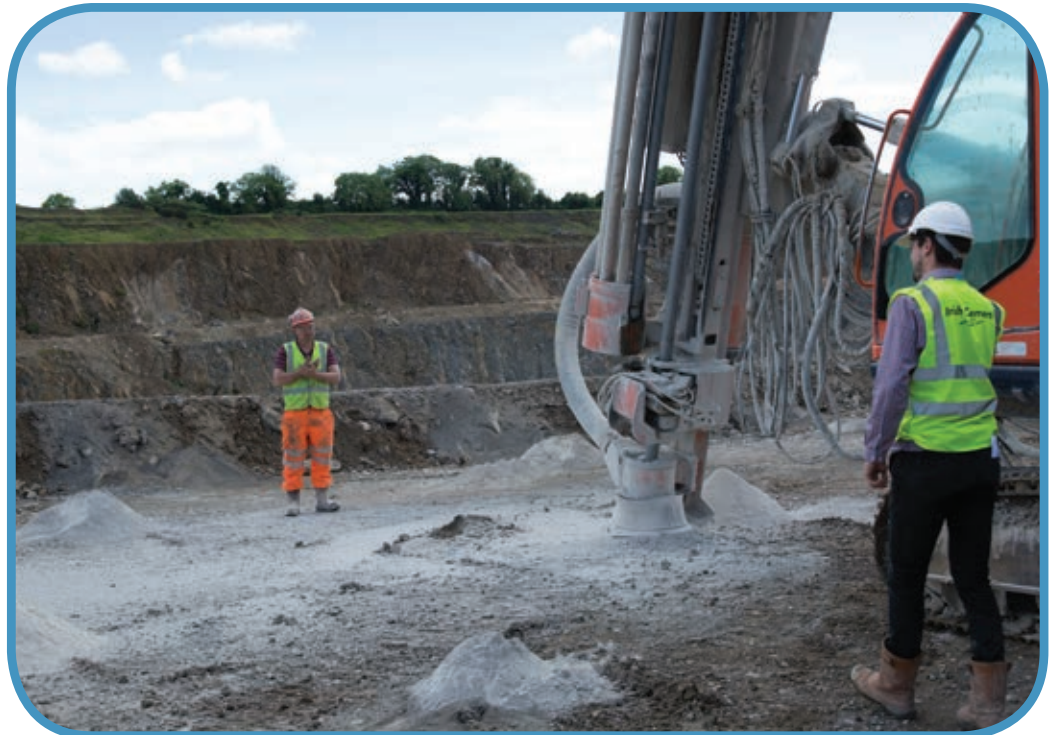
Quarry Workers marking out drill holes with fall protection provided by bunded edge protection made from quarried material
