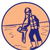
Before the ground is broken, the area should be scanned with a detector to verify the position of any services. Any variations identified should be noted on the drawings. The position of the service must be carefully marked, to ensure that subsequent work does not come into contact with it.
