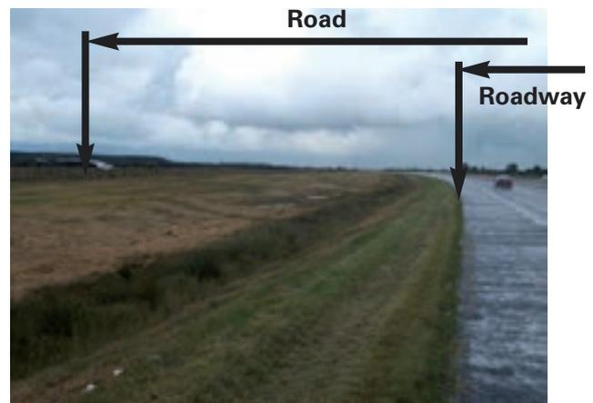
**Photograph 2** Section of carriageway showing how the road can extend way beyond the roadway.
