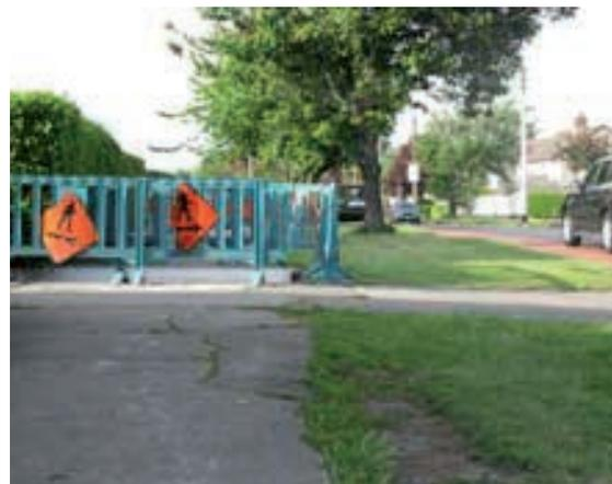
*Photograph 12* Construction work on footway; access around the footway for users is on the grass margin a safe distance from the roadway.
