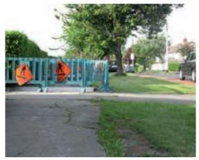
**Photograph 12** Construction work on footway; access around the footway for users is on the grass margin a safe distance from the roadway.
