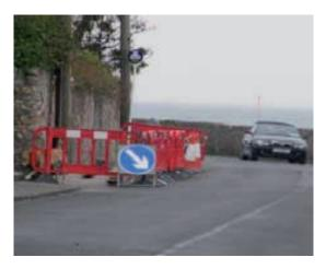
**Photograph 8** Footway closed at busy bend; no alternative provided for users to pass construction work. No safe access to or from bus stop.
