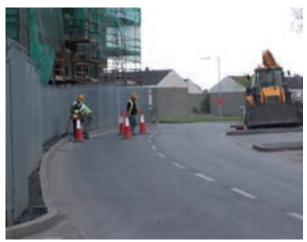
**Example 2** Three workers carrying out construction work at busy bend on roadway. Insufficient and inadequate signing, lighting and guarding measures in place to protect the work crew and other road users.
