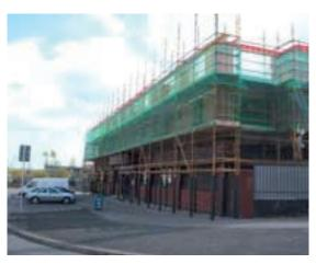
Photograph 11 Scaffold erected on a wide footway.
