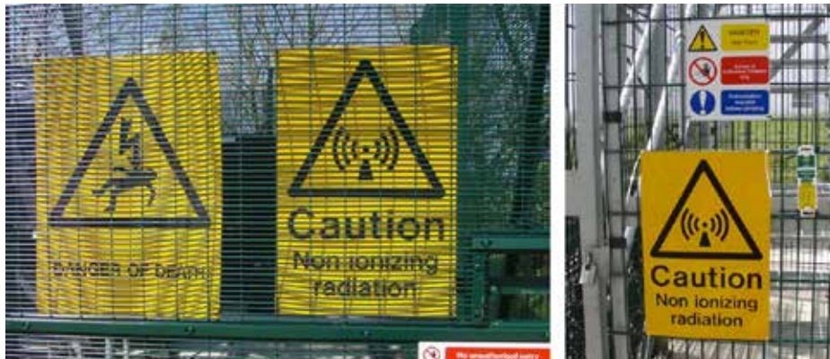
Figure 12.4 — Warning notices on the gate to the radar compound (left) and on the gate to the antenna tower (right)
