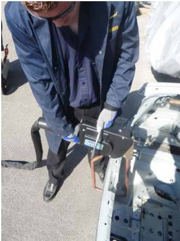
Figure 6.1 — A hand-held spot welder being used to fix a new panel in place
