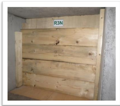
Regulator in tunnel complex
