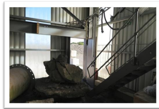
#4 Crusher – View towards access
