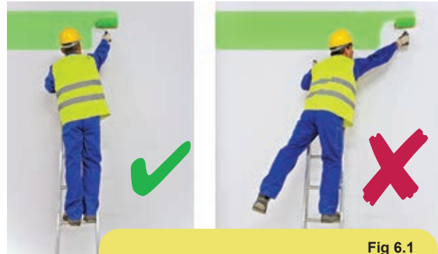
Fig 6.1 Maintenance work involving work at height
