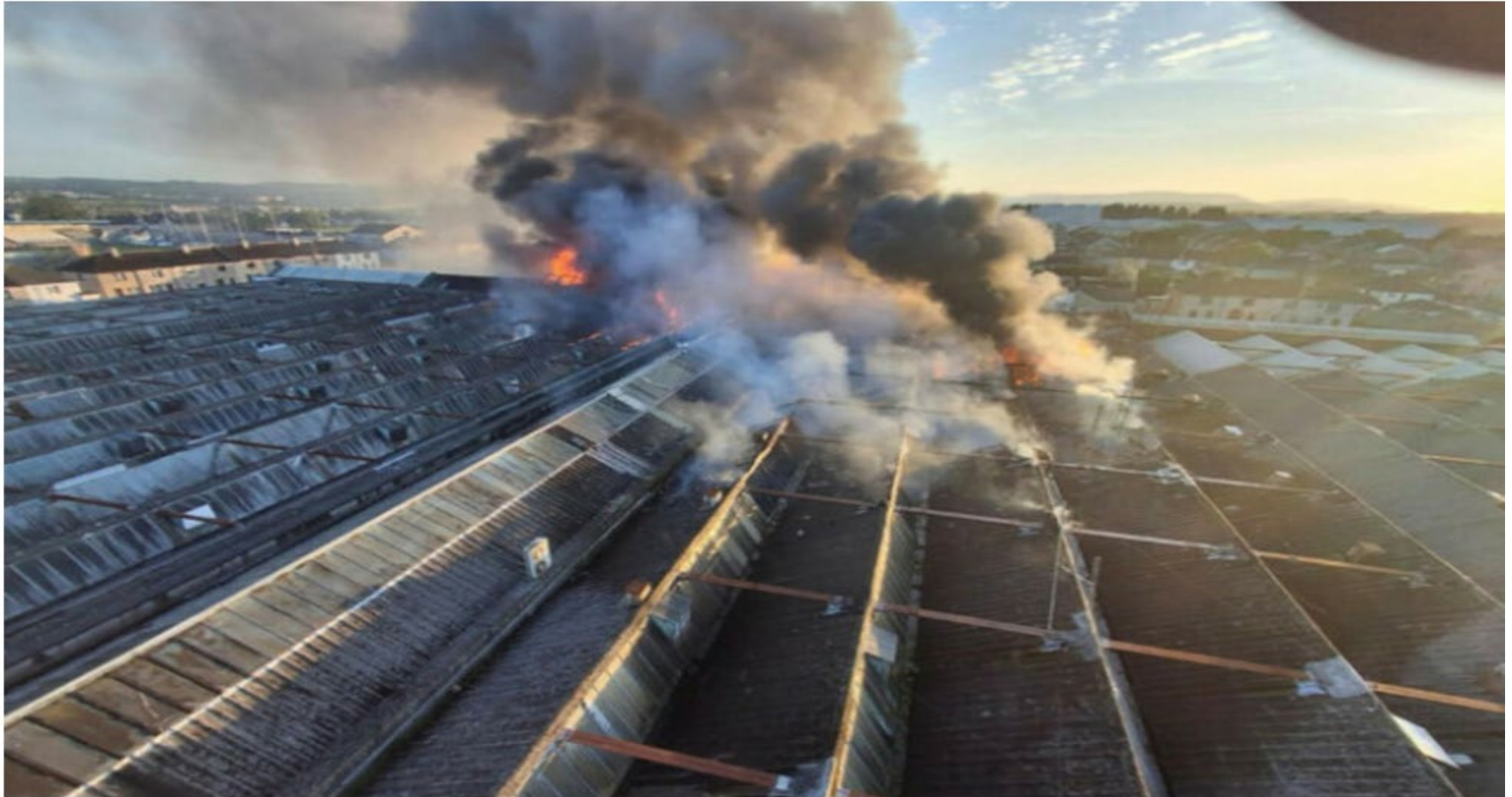
Aerial image of the fire. IMAGE: Waterford City and County Council
